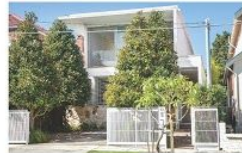
39 Hendy Avenue South Coogee
